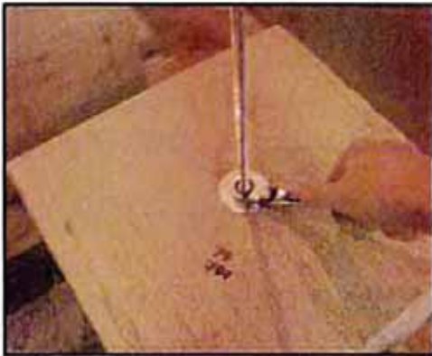
(c) Rod Stabilization (2"OD -3/8"ID Washer & Nut)
