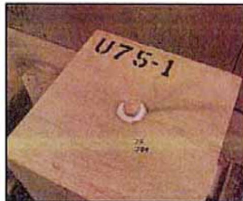
(f) Insertion of Insulation around the Rod (Silicon added to Seal the Hole)
