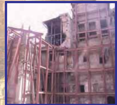
Structures with temporary supports
