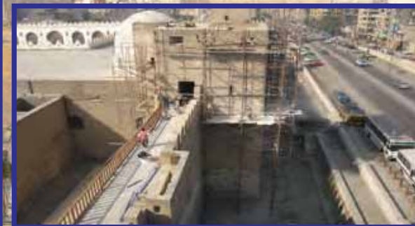
Structures with temporary supports
