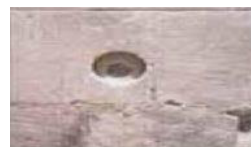
Anchor installed & inflated ready for front core to be replaced.
