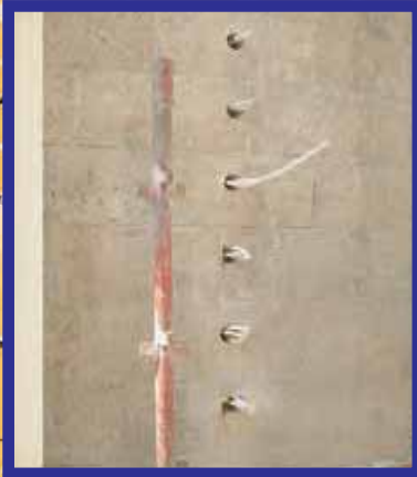
Internal cross walls stitched and secured to the external walls.
