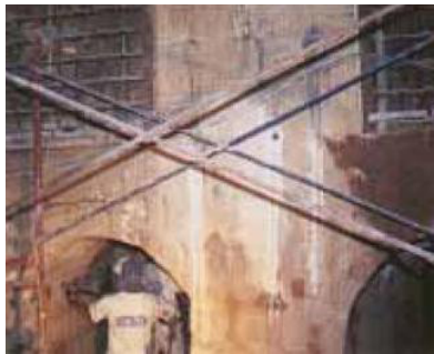
Drilling the vaults.
