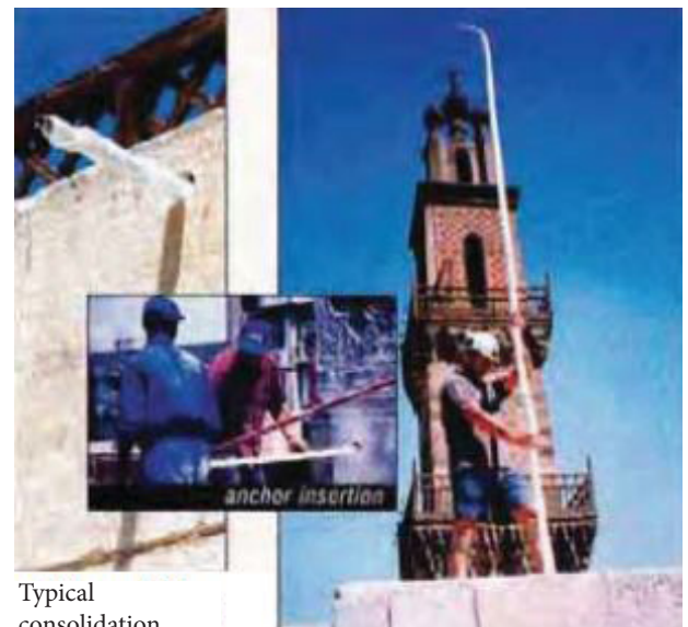
5 meter long vertical anchors at roof level
