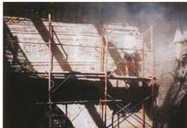
Decorative panels being drilled ready for installation of consolidation anchors.
