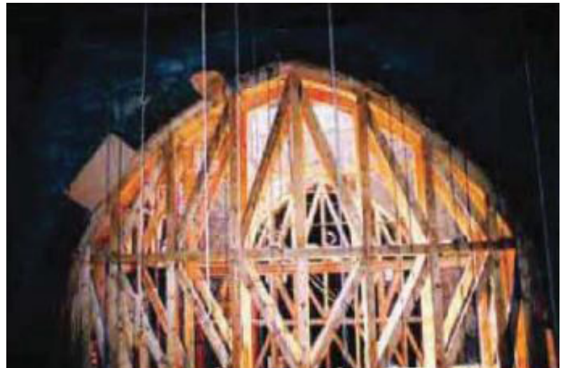
Temporary support of the Dikka arches
