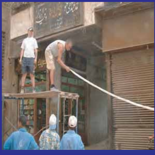
Positioning anchors in confined areas
