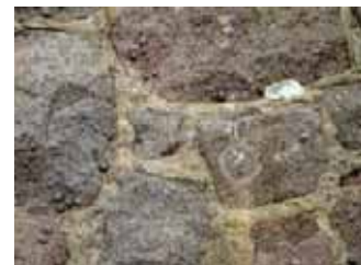
Figure 20 - Anchor with plug cap replaced, 'Secret Fix'
