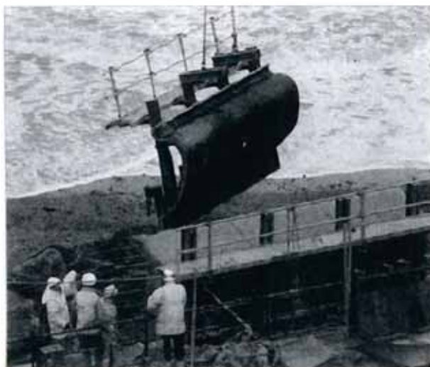
Figure 4. Typical shape of 'recurve' from Ciria C674 (Dupray et al. , 2010)
