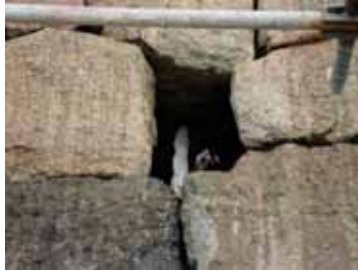
Figure 16 - Pre-injection with masking tape
