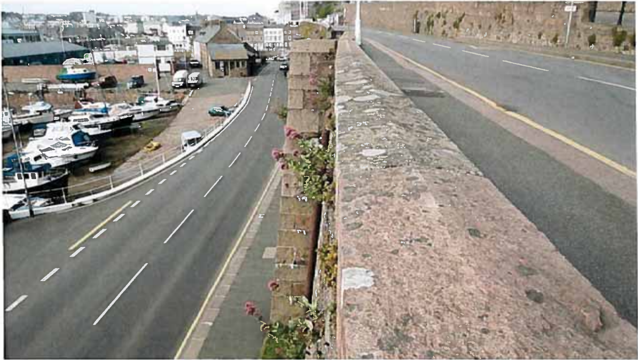
Fig 5 View looking up
