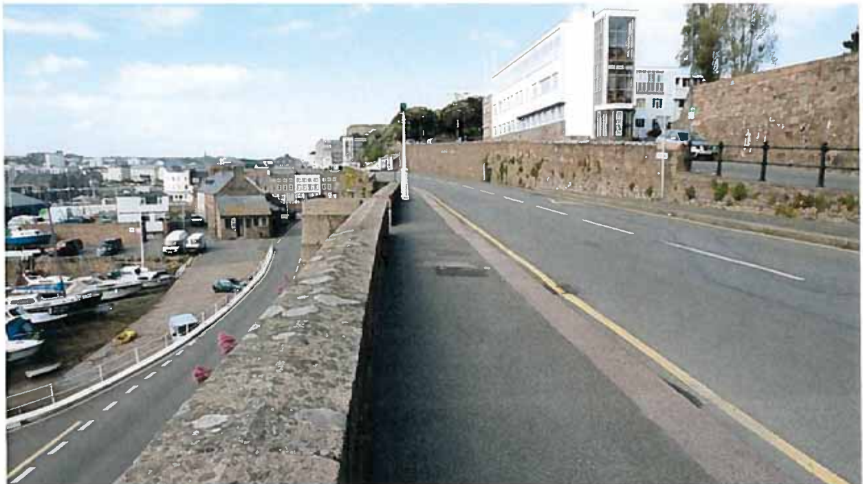
Fig 4. View looking up
