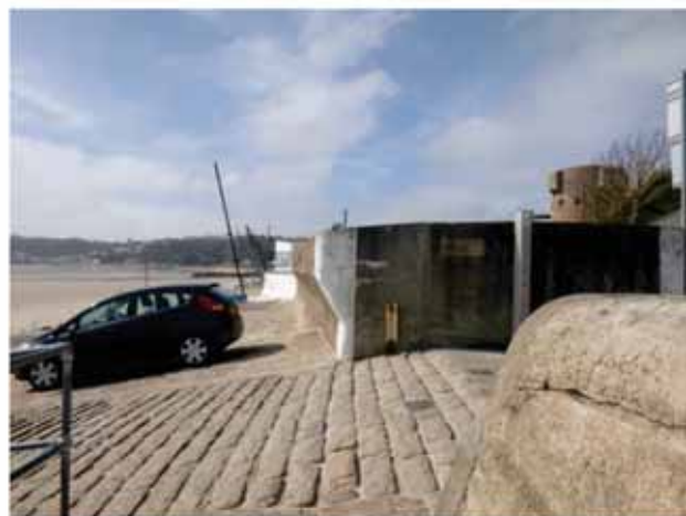
Figure 9. Gunsite angular recurve at the slipway
