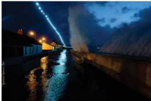
Figure 15. Storm wave action at new wave return wall and existing
