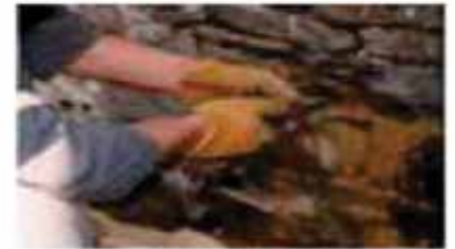
Insertion of 3m Cintec Anchor (left). Its inflation using cementitious grout, (above).
