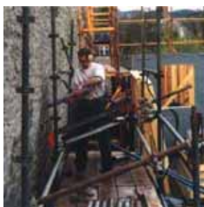
Extracting the tube liner
