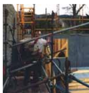
Removing the tube liner
