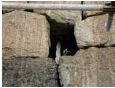
Pre-injection with masking tape
