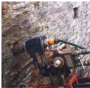
Drill head at full depth
