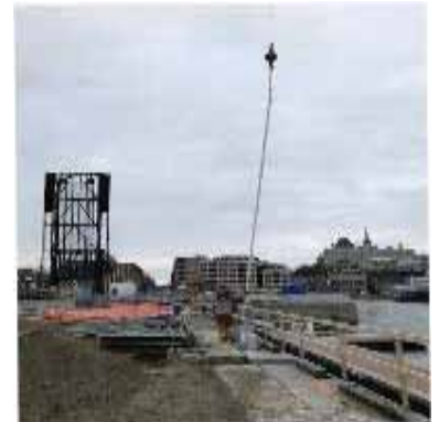
Cintec anchors being lifted into place Quebec Canada
