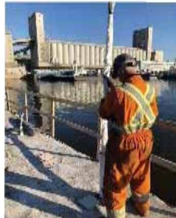
Cintec anchors being placed by installer
