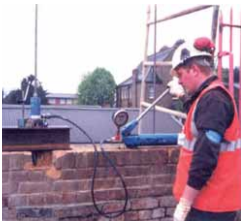
Post-tensioning Cintec anchor in test panel.
