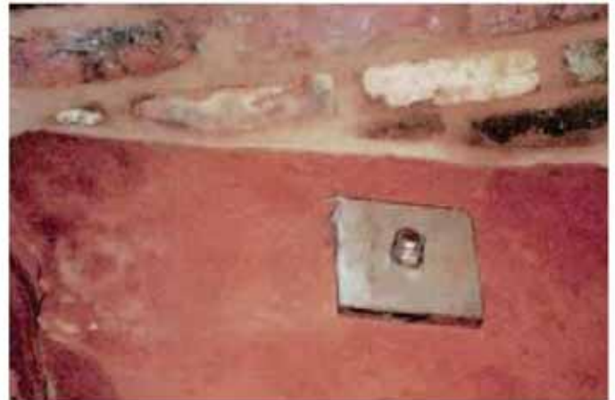
Roof bolt support to ballroom ceiling.
