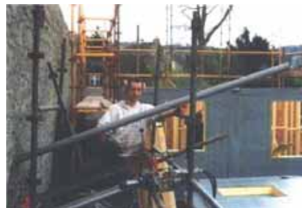
Inserting plastic tube liner to the drilled hole
