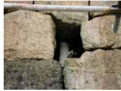
Anchor grouted & expanded
