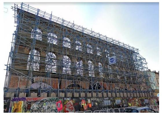
The building had remained in a very poor neglected and derelict condition for over 35 years and during the past few years a design scaffolding had to be erected to provide support to the listed facade as some buildings behind were becoming dangerous.
