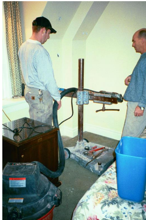
Dust – free Directional Drilling
