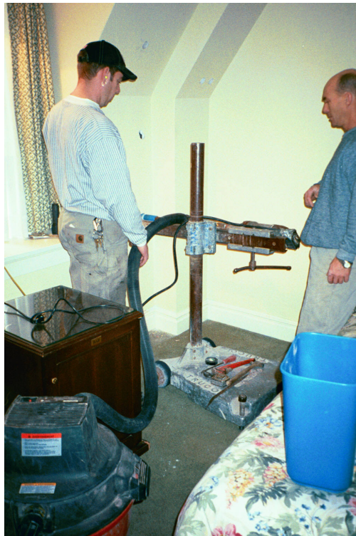
Dust – free Directional Drilling
