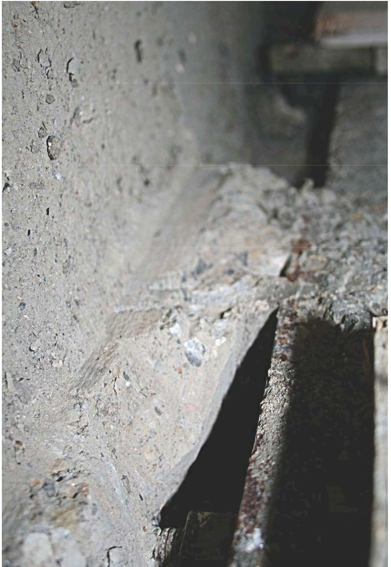
Internal end of the precast concrete beam. Photograph 16
