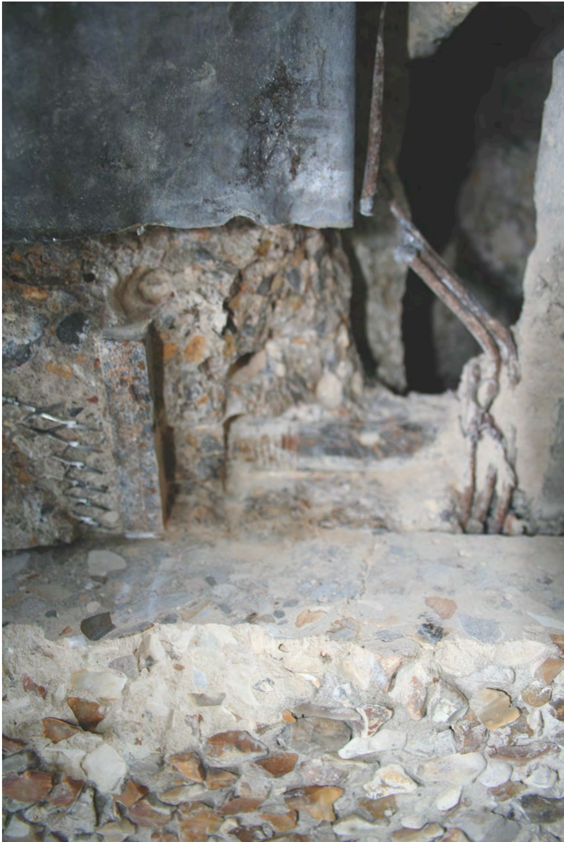
Original wall connecting bolt.
