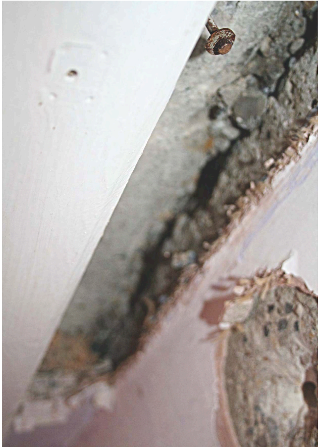
Floor slab to wall connection viewed from below. Photograph 11
