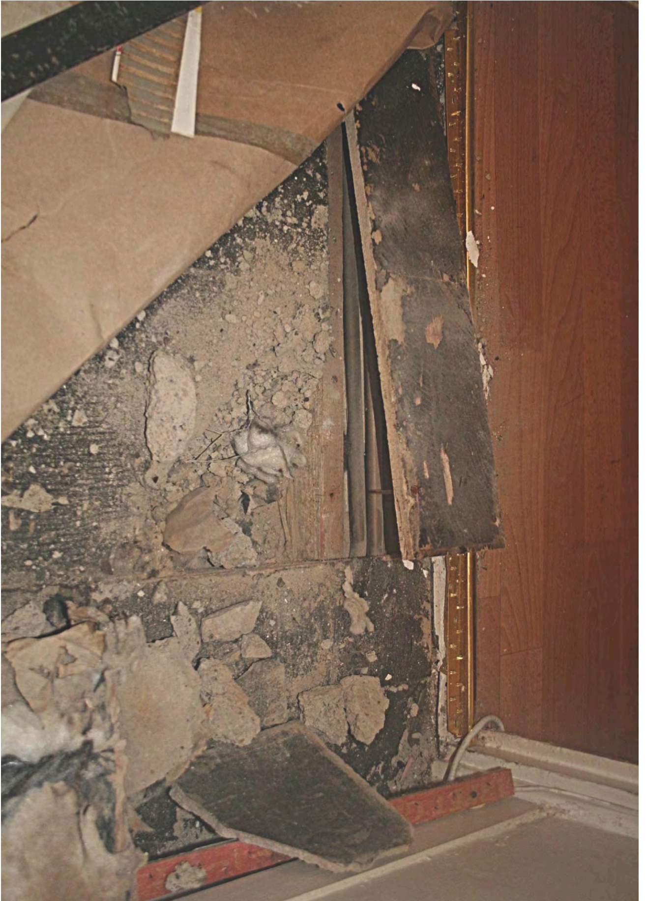
Water pipes exposed adjacent to wall. Photograph 15
