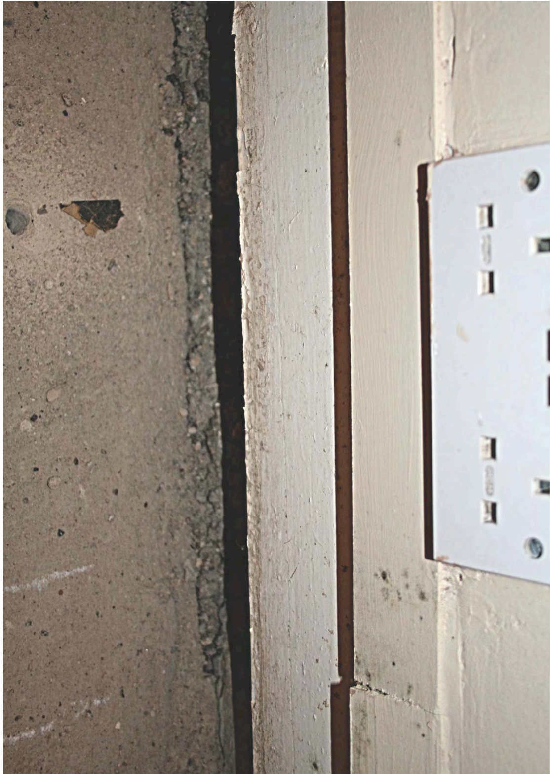
Floor slab to wall connection viewed from above. Photograph 12
