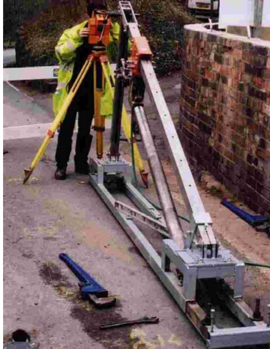
Figure 2.2 Installation using Precisely Aligned Diamond Drilling Coring Equipment
