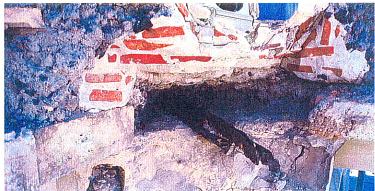
Once the cornice had been partially disassembled, the materials and techniques used in its construction could be easily identified. Note the clinker concrete, or "cindercrete," between the terra-cotta blocks and the brick backup material, and the severe deterioration of the steel supports. CSI recommended that all new steelwork be AISI Type 316 stainless steel, a non-corroding type, which is essential in this chloride-rich maritime environment.
