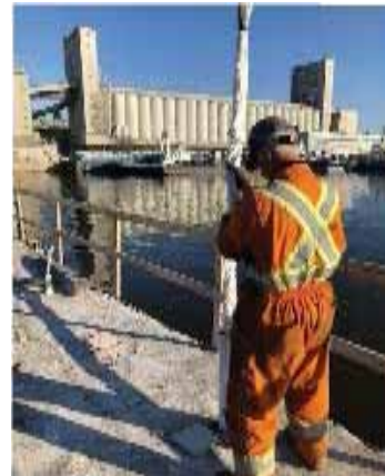
Cintec anchors being placed by installer
