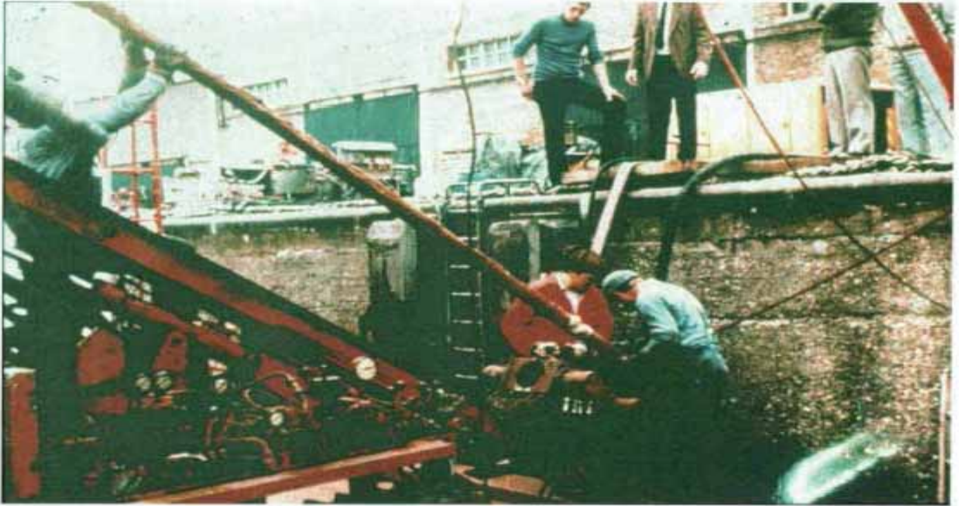
Strengthening of Zeebrugge Harbour Wall (Belgium)
