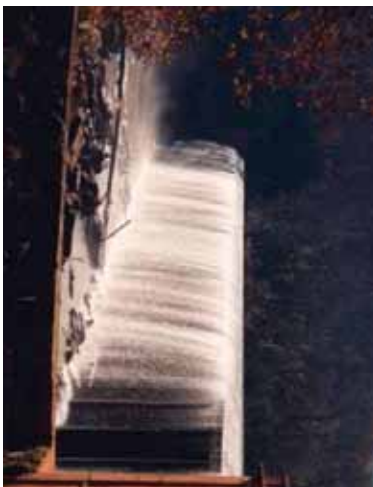
Georgia-Power Bartletts ferry dam, Athens, Georgia, USA
