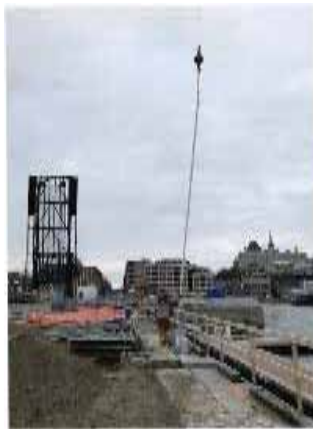
Cintec anchors hoisted into place by crane
