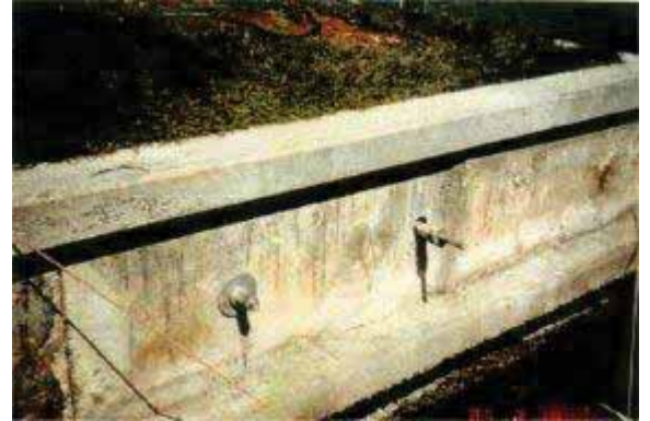
Florida Sea Wall - Subsidence & Dislocation
