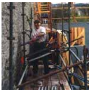
Extracting the tube liner
