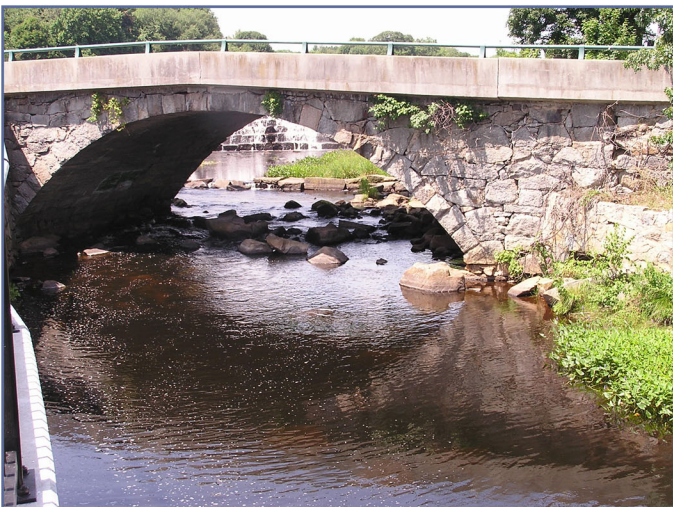
Harrisville Bridge, Harrisville, NH
