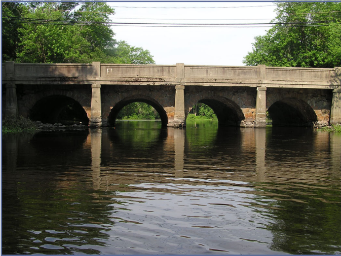
Ames St. Bridge, Dedham, MA
