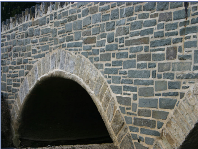
Century Lane Bridge, Buck's County, PA
