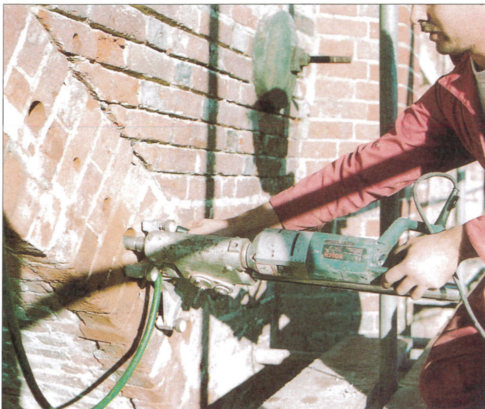
Core drilling holes for the anchors
