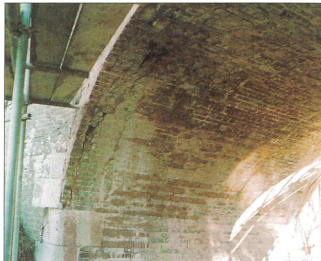
Typical damage to the soffit of the bridge
