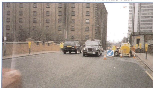
DUCIE BRIDGE - MANCHESTER
