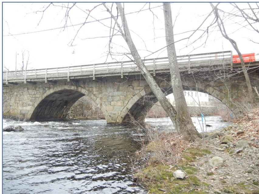
Slattersville Bridge, North Smithfield, RI
