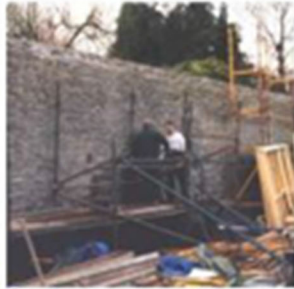
Setting up the drilling rig
