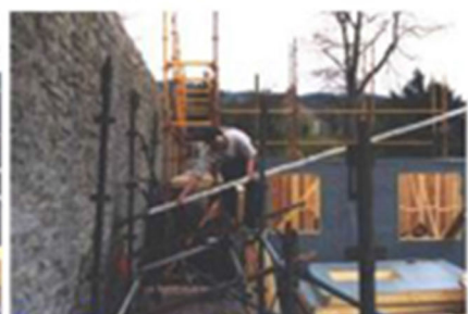
Carefully placing the anchor
