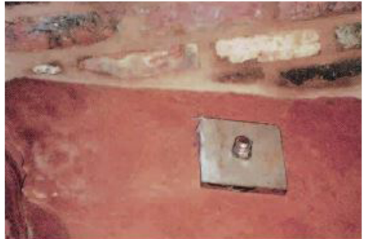
Roof bolt support to ballroom ceiling.
