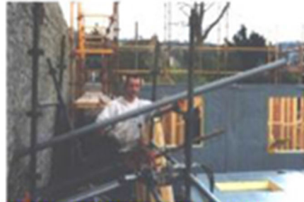
Inserting plastic tube liner to the drilled hole
