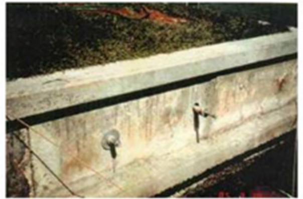
Florida Sea Wall - Subsidence & Dislocation
