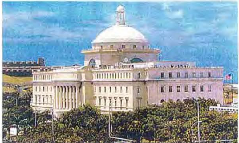
Puerto Rico's Capitol Building, or "El Capitolio," in San Juan, was completed and inaugurated in 1929. A major port city, San Juan faces the Atlantic Ocean to the north. This marine environment was a major factor in the dangerous corrosion of the anchoring system of the building's terra-cotta cornice.
