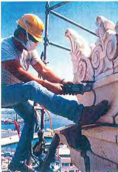
A worker is seen here cutting the mortar joints between the terra-cotta blocks in preparation for the disassembly of the cornice.
