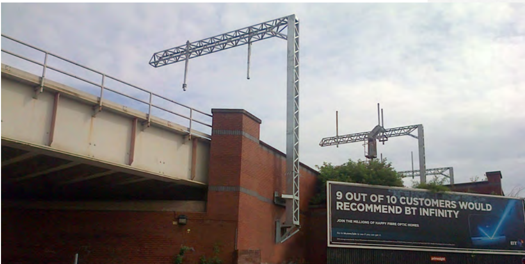
Twin Track Cantilever Portal. Installed with 11m long Anchors drilled right through bridge to other side.
