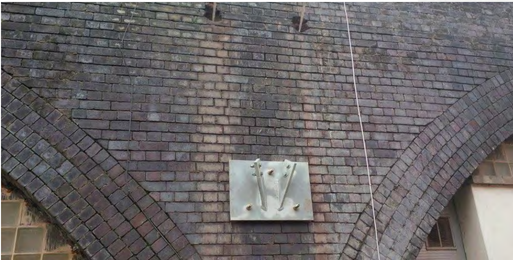
6m long Cintec Anchors installed at 45 degrees
