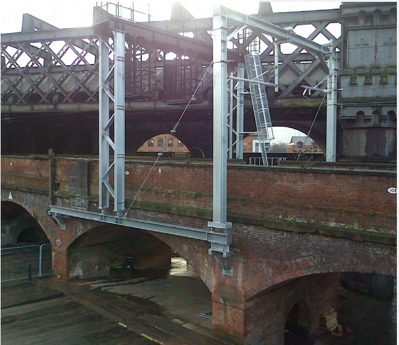
Combined electric and signal gantry.
