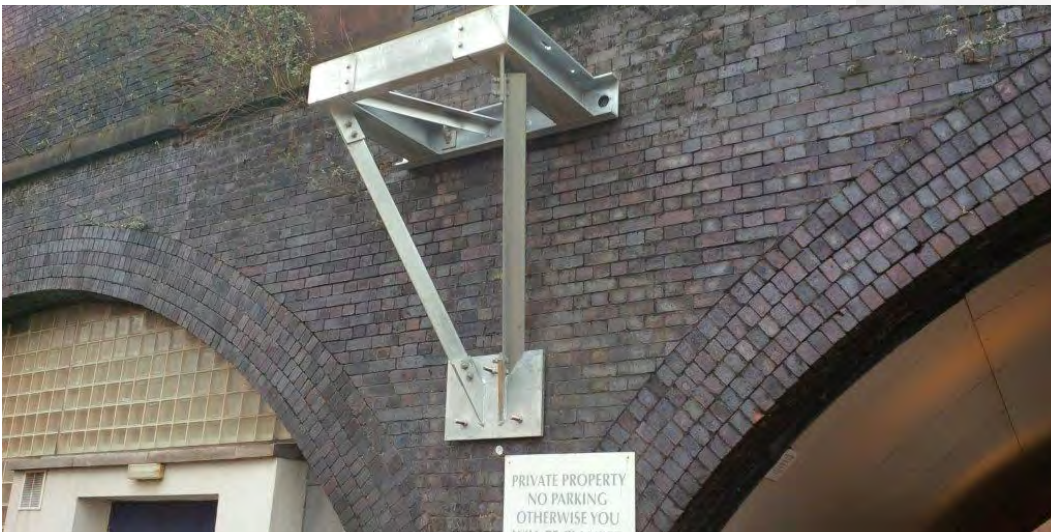
Solid blue engineering brick construction
