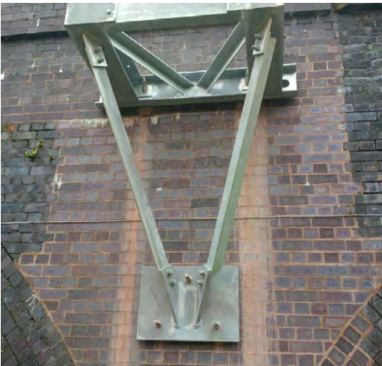
Smaller horizontal anchors for the base plate.
