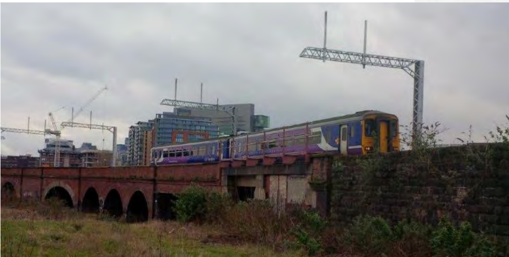
General view. Note: Work carried out whilst line was live.
