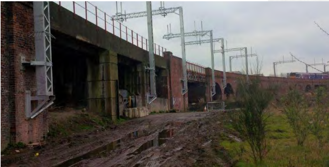
Work carried out in open and messy site conditions.
