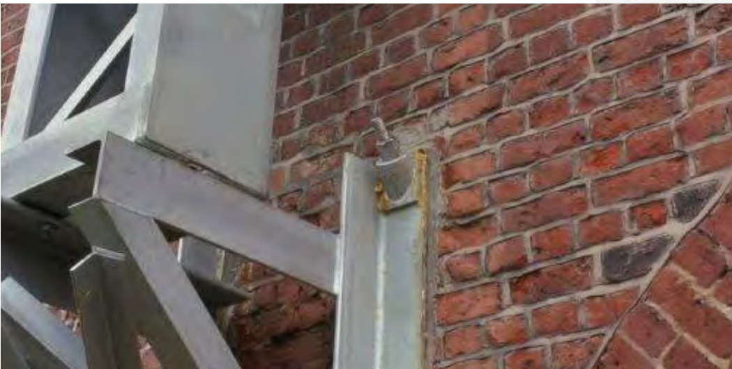
Close up of 45 degrees washers and locking nuts.
