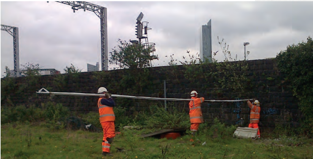
Inserting the Anchor - 11m in length.
