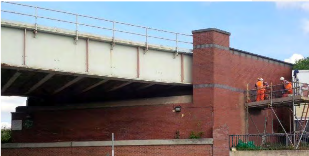
Three off 65mm diameter holes at 11m.
