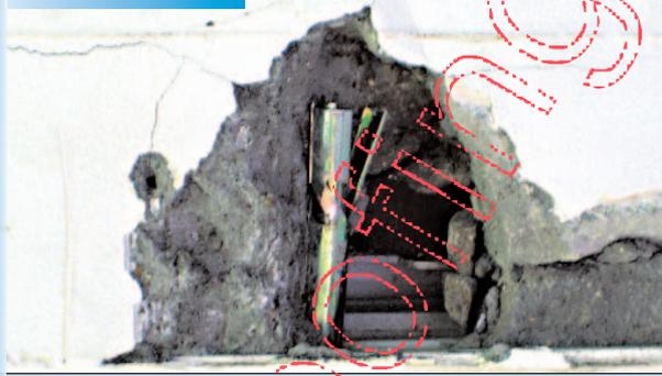
Figure 3 Door Perimeter Spalling
