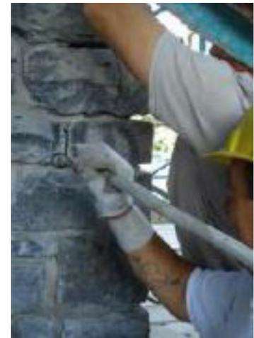
The stabilization of the East wall corners and the stabilization and stitching of the East and North walls was carried out by masonry contractor DeMarinis (DMA) Inc (Tony DeMarinis, President.). DeMarinis had used the Cintec system for almost 20 years, on several projects, and was therefore very knowledgeable on its ease of use and capabilities. In this case, over 1,000 Cintec anchors were installed in lengths from 21 inches to over 15 feet long.
