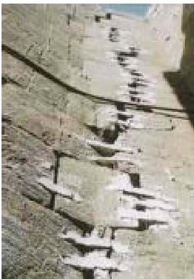
Vertical shear crack
