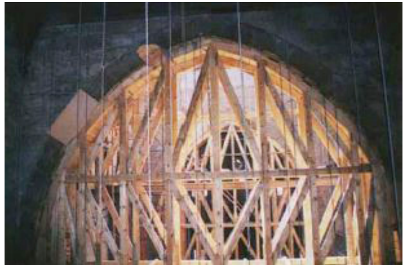
Temporary support of the Dikka arches
