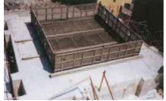
Roof section above central courtyard
