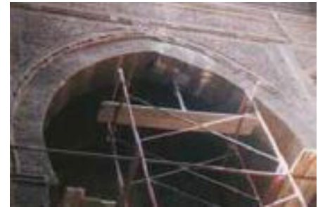
One of the four arches of the court being scaffolded prior to drilling and anchoring.
