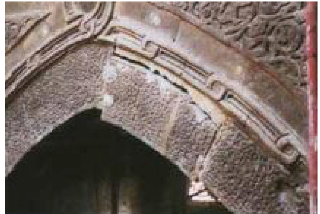
Seismic damage to decorative arches
