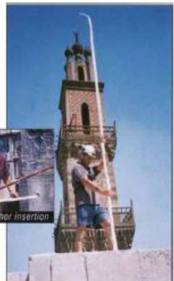
5 meter long vertical anchors at roof level
