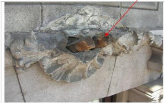
View of location where Loose ornament was removed. Wood block s = 10", embedment of wood blocks = 5-1/2"
