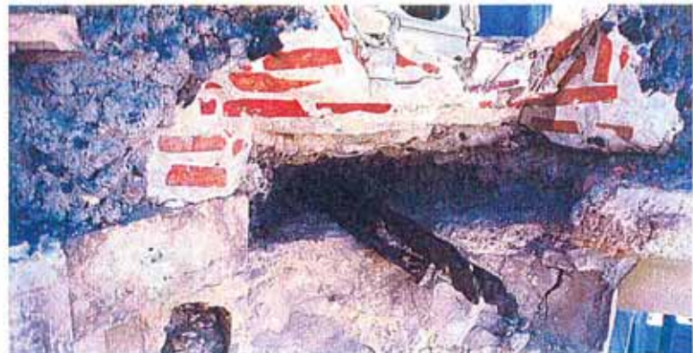
Once the cornice had been partially disassembled, the materials and techniques used in its construction could be easily identified. Note the clinker concrete, or "cinderente," between the terra-cotta blocks and the brick hachup material, and the severe deterioration of the steel supports. CSI recommended that all new steelwork be AISI Type 316 stainless steel, a non-corroding type, which is essential in this chloride-rich maritime environment.
