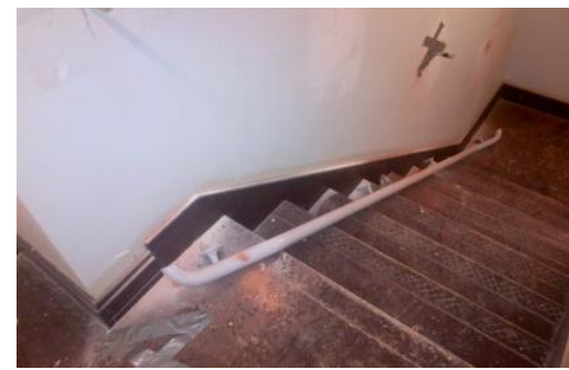
Two of the four anchors installed in the wall, note the exposed thread for attaching the handrail.
