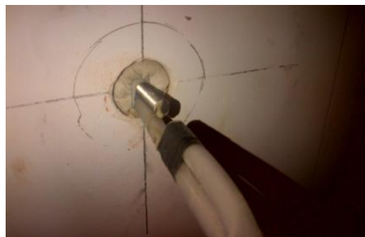
Installed anchor in the wall
