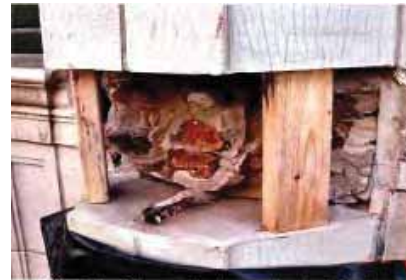
Fig. 2 - Corroded restraint fixing
