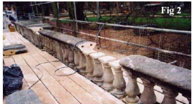
Holes drilled horizontally through the parapet.
