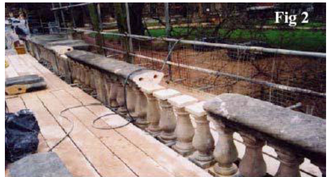
Holes drilled horizontally through the parapet.
