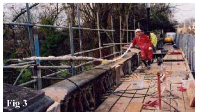
Shows a horizontal Cintec anchor prior to installation.
