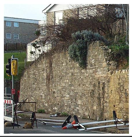
As can be clearly seen in the photograph to the left a horizontal fracture had developed in the wall approximately one metre above pavement level with the wall above trying to "fold" at that point due to the forces of the retained ground.
