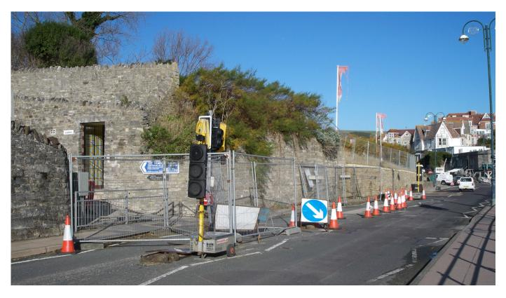
In 2008 Dorset County Council contacted Cintec International Ltd to ask them to submit a solution to an already structurally failing retaining wall on the main sea front road in the town of Swanage. To ensure public safety without a total blockade of the highly trafficked road a traffic management system and barricades had been installed before Cintec visited the site.
