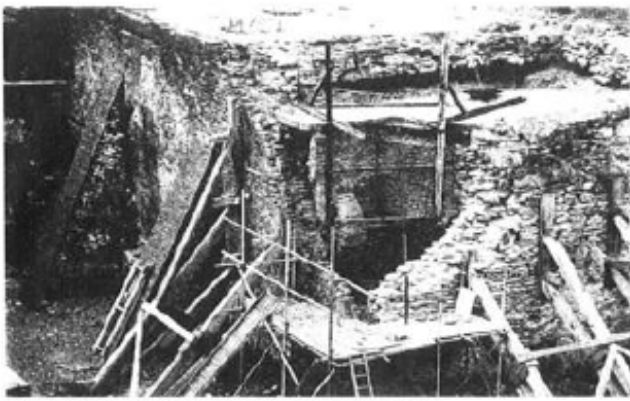
Fig 5. Southeast corner excavated prior to rebuilding
