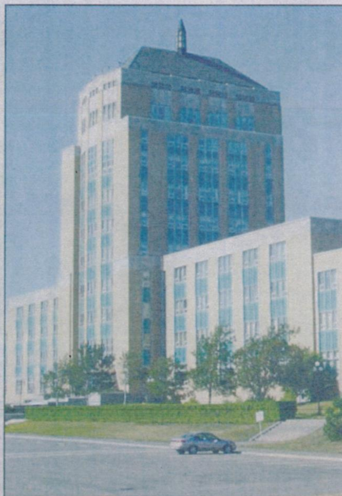
PROJECT: Staff from Cintec have been called in to work on this prominent government building in Canada to make it secure
