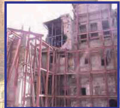
Structures with temporary supports
