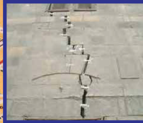
Typical damage caused to exterior walls
