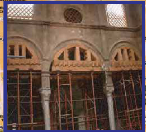
Buckling and movement of columns
