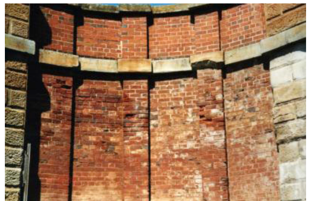
Damage to wingfall – note coloured cement render from 1930's and salt deposition caused by it.
