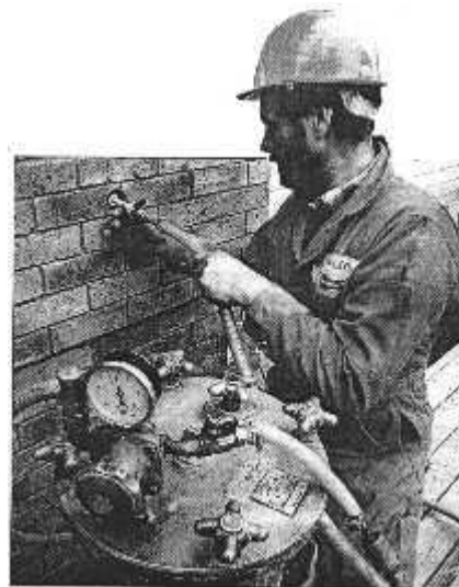
...then insert the tubular ties and pump in the grout.
