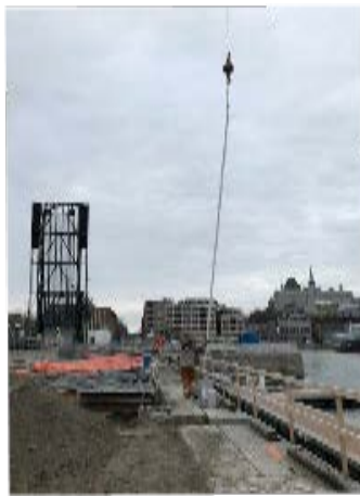
Cintec anchors hoisted into place by crane
