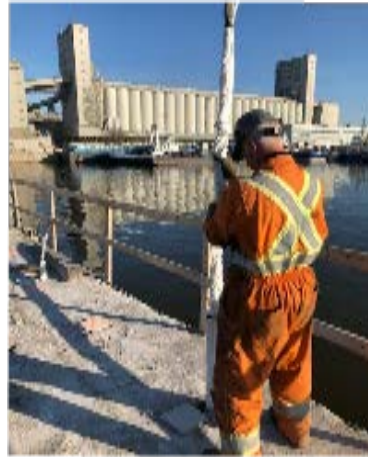
Cintec anchors being placed by installer
