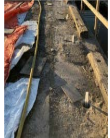
Cintec anchors in place prior to inflation
