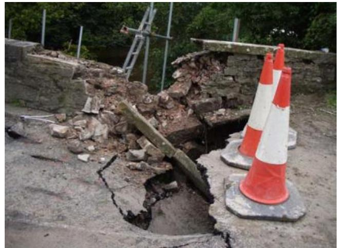
The damage to the upstream spandrel and parapet was mainly limited to the large area of damage above the west abutment and a significant crack above the east abutment. Damage to the downstream spandrel and parapet was more widespread, with cracking through mortar joints almost throughout the length of the wall.
