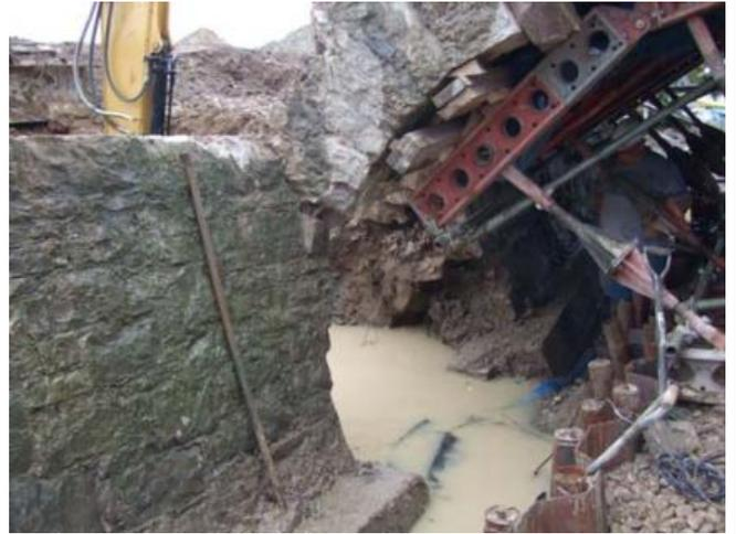
The flood had caused the abutment to move which necessitated the complete removal of the abutment and providing a new foundation and concrete abutment, which was subsequently faced with stone.
