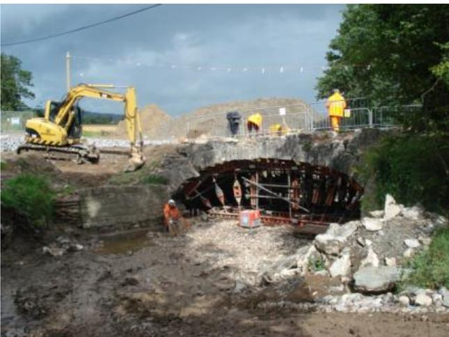
New culvert installed to act as a permanent flood relief system which was put to the test shortly after the project was completed.
