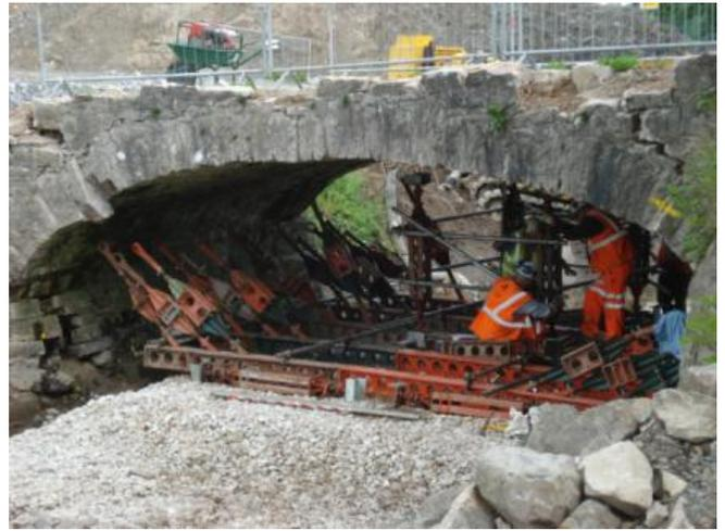
The arch was propped underneath and the parapet walls removed.
