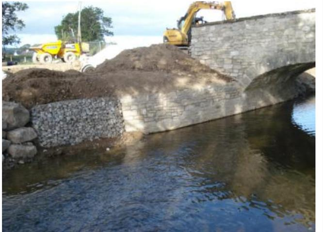
New gabions were placed to protect the river bank and training walls constructed, faced with stone to match the structure.
