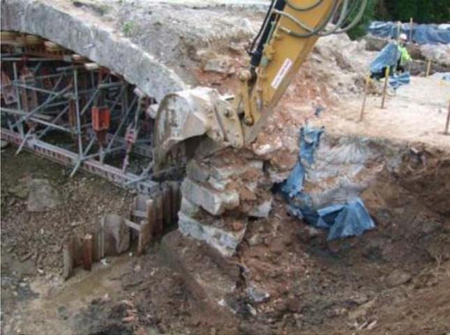
After the installation of the Cintec anchors to bring the bridge back to a 40 tonne capacity, the roadway was reconstructed to the original profile.
