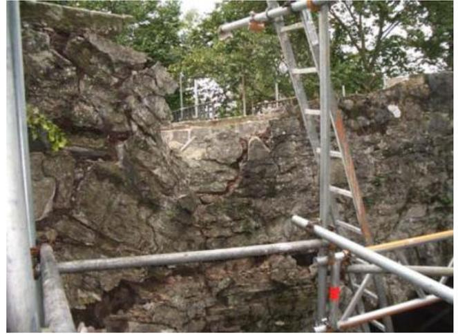
The movement of the road surface suggested that the arch barrel had rotated up to 4.5 degrees about the east springing. There was distortion of the arch barrel due to differential movement, resulting in a shear crack at the west upstream corner. The fact that this corner is lower than the adjacent arch barrel suggested that the abutment dropped vertically at this corner, followed by the adjacent arch barrel. Apart from this south west corner, the arch barrel was in reasonable condition.
