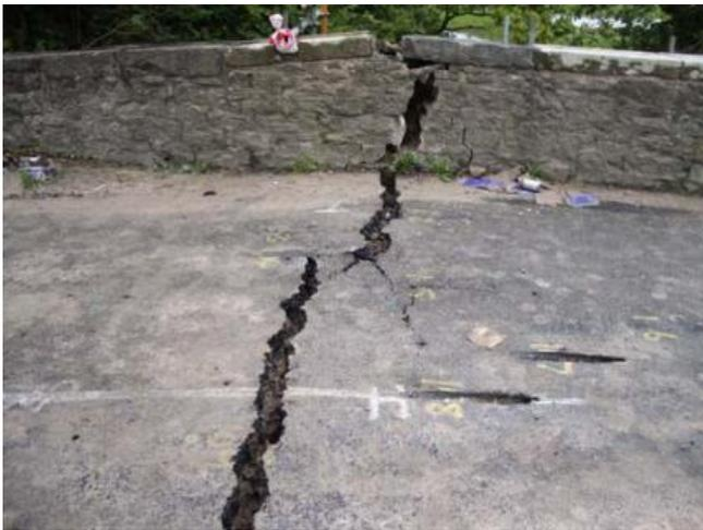
The east abutment appeared to be intact with no movement or cracking identified. The west abutment appeared to be intact at the upstream elevation. At the downstream elevation there was a large amount of dilatency of the masonry, with severe cracking and evidence of movement on both faces.
