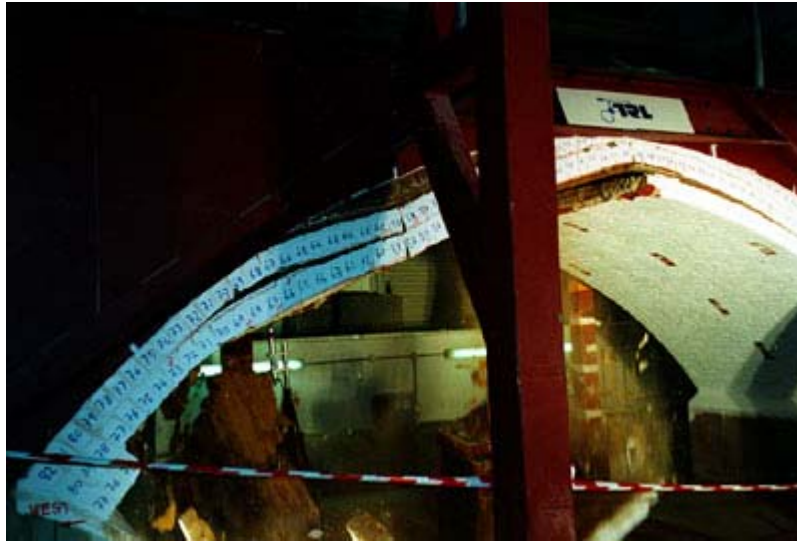
Figure 3 Collapse of Strengthened Arch
