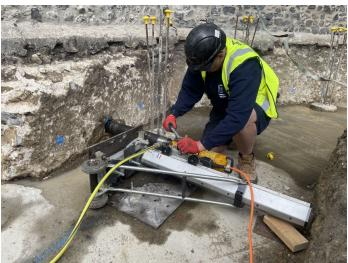
24mm diameter stainless steel Cintec anchors in 100mm diamond core drilled holes were set at 600mm horizontal centres into the side of the flint/mortar foundation. These would effectively transfer the 95kN shear load to the piles.
