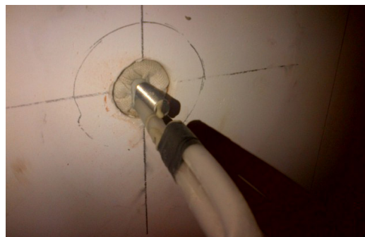
Installed anchor in the wall
