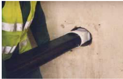
Insertion of Cintec anchor section of 'I' beam into brickwork.
