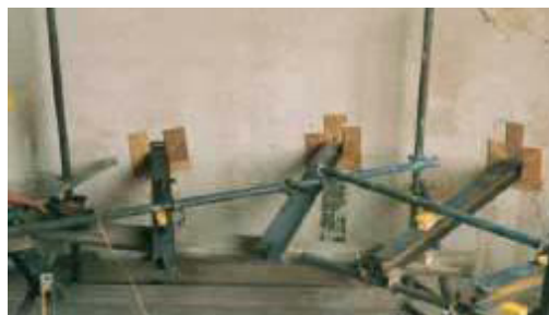
All installed 'I' beams levelled and supported as grout Hardens.
