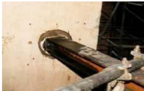
'I' beam following anchor grout injection.
