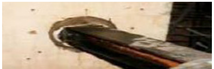
'I' beam following anchor grout injection.
