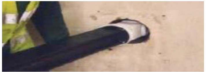
Insertion of Cintec anchor section of 'I' beam into brickwork.
