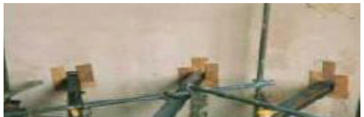
All installed 'I' beams leveled and supported as grout Hardens.
