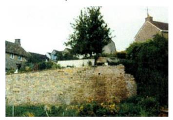
In order to maintain the structural integrity of the wall, English Heritage advised the specification of Cintec ground anchors for a number of phases for the work. Stability was returned to the wall by inserting Cintec ground anchors through the thickness of the wall and into the clay and limestone behind.
