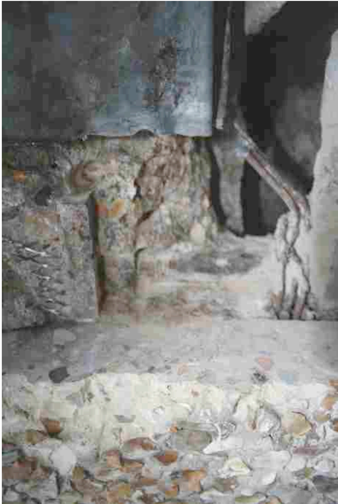
Original wall connecting bolt.
