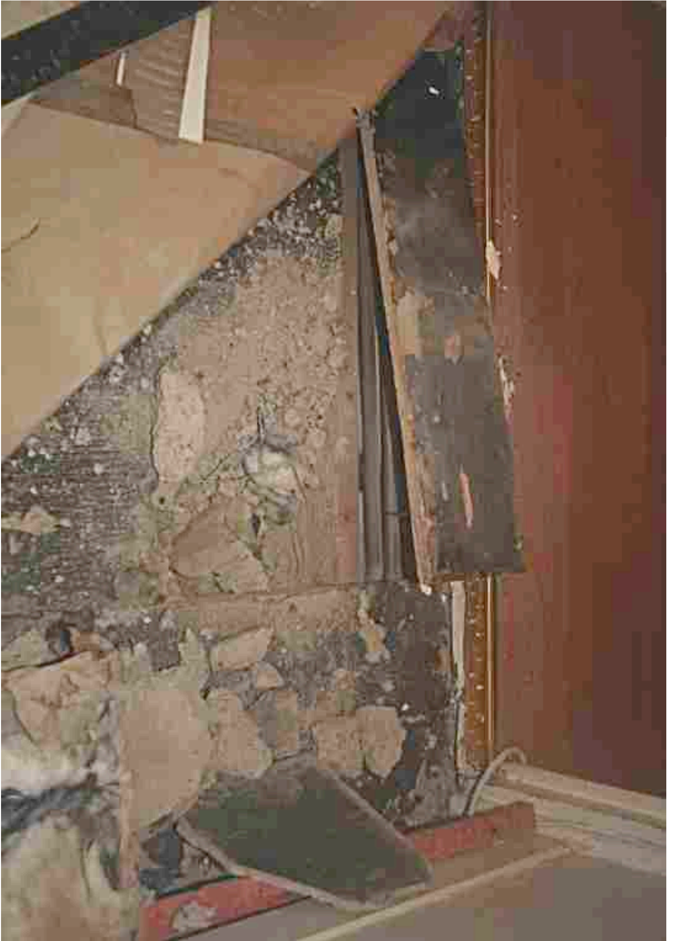
Water pipes exposed adjacent to wall. Photograph 15
