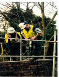
Finally the sandstone parapet coping stones were replaced and two missing stones reproduced. The solution provided the necessary increase in wall strength without having any visible change to its appearance.
