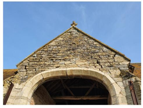
The structural integrity of one of the main arches above one of the main entrances had been compromised by settlement and rotation of left hand return wall due to older alterations to the adjacent ground.
