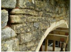
Temporary timber propping was in place to support the failing arch while the installation of anchors was carried out.
