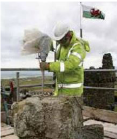
Diamond drilling to install anchors to secure stonework to high level chimney stack.
