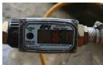
Flow meter measuring water in bag.
