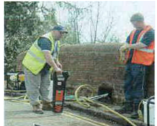
Checking for sub-surface services during bridge survey.
