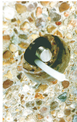
Injecting grout into anchor.
