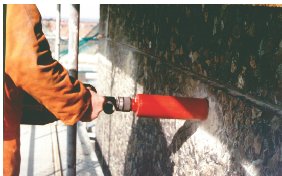
Diamond core drilling.
