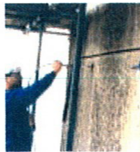
Injecting grout into anchor.
