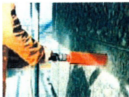
Diamond core drilling.
