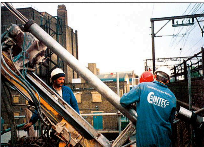
The assembling and installation of a compression anchor
