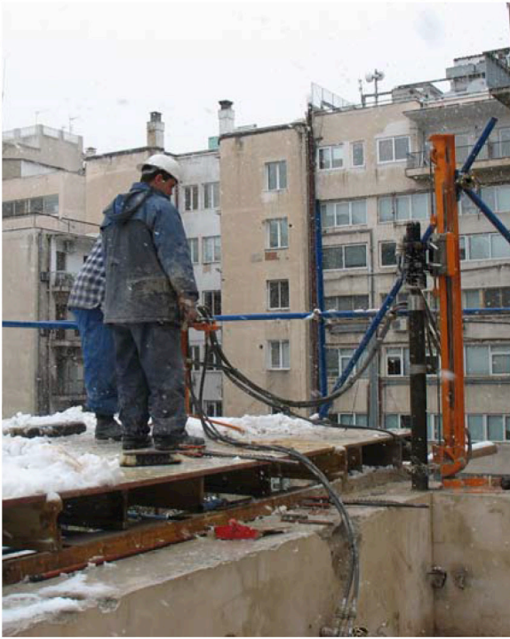
Vertical holes dry diamond drilled.
