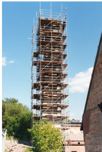
Chimney Restoration In Progress
