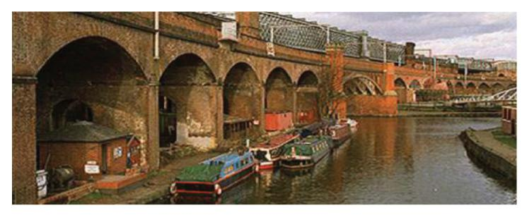
The busy Deansgate rail viaduct is situated in the heart of Manchester spaning numerous buildings, roads and canals. In 1997 the normal daily flow of railtraffic was disrupted by a destructive fire which took hold in a workshop located directly underneath. The subsequent heat generated by the blaze caused extensive damage and a weakening of the seven rings of masonry that form the arch barrels. The surface ring of brickwork completely delaminated and collapsed to the ground below.
