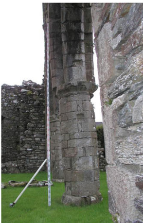
Image revealing the extent of wall and column rotation prior to stabilisation
