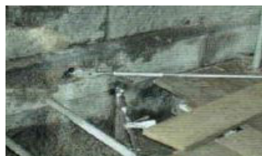
Lower fixing detail with turn buckles.
