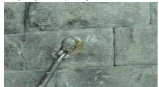
Upper Fixing Detail - Cintec Stud Anchor with Eye Nut attachment.
