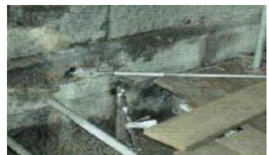
Lower fixing detail with turn buckles.
